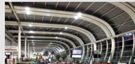
Metal ceiling, airport, India
