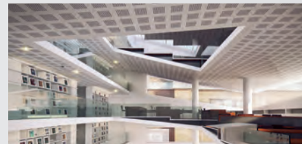
Plasterboard ceiling, library, Spain
